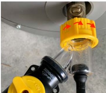
Hand Tighten to drain valve
