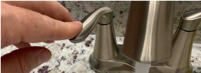
Hot Water Faucet turned on, leave on until step 11
