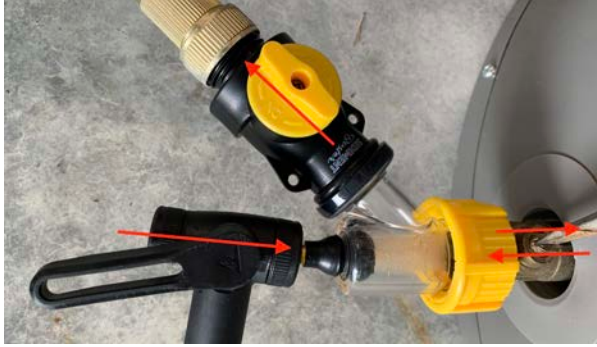
Both Sediment Buster™ and Drain valve open
