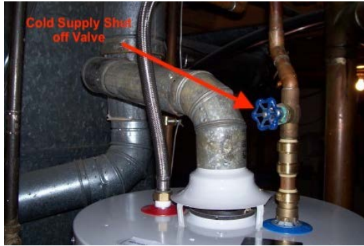
Gate Valve, Rotate Several Times
