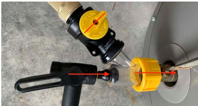
Drain Valve open, Sediment Buster™ Valve Still Closed
